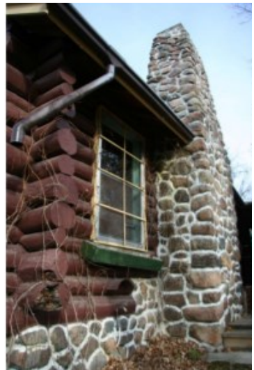
Saddle Notch construction detail
